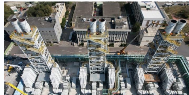
Taipower Tunghsiao Power Plant Renewal program
